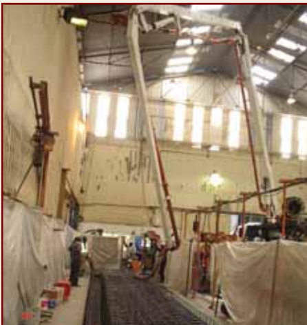
Pouring of concrete
